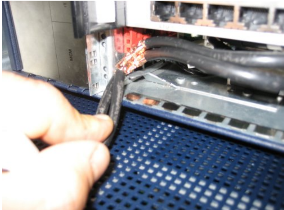
Figure 50: Cavo DC staccato
