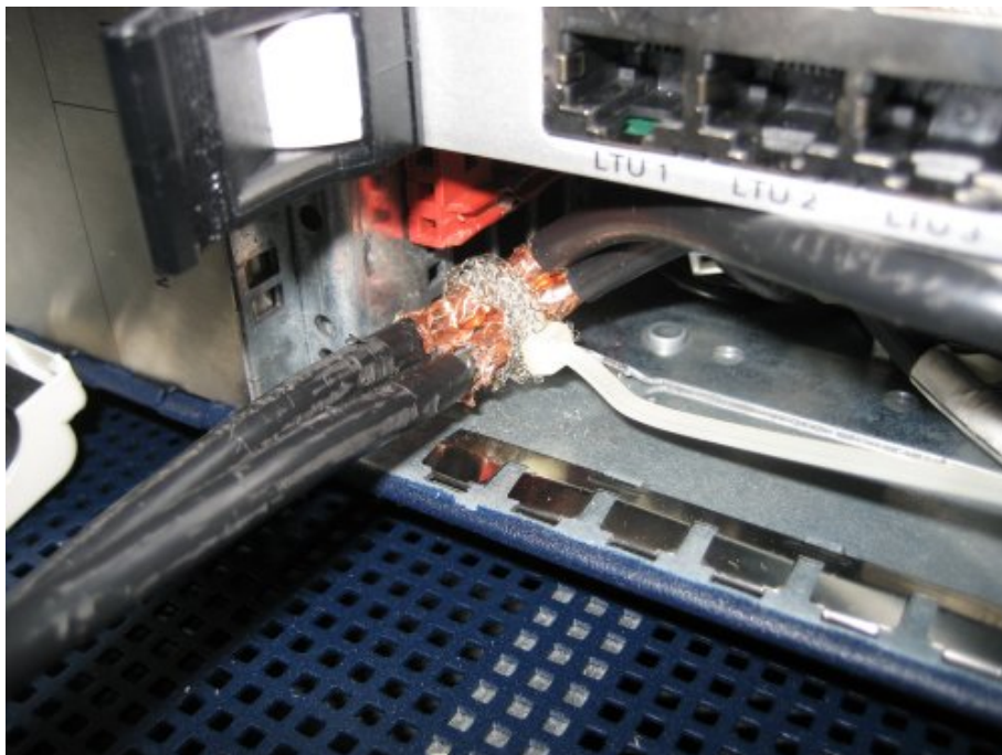
Figure 44: DC cable shield on housing
