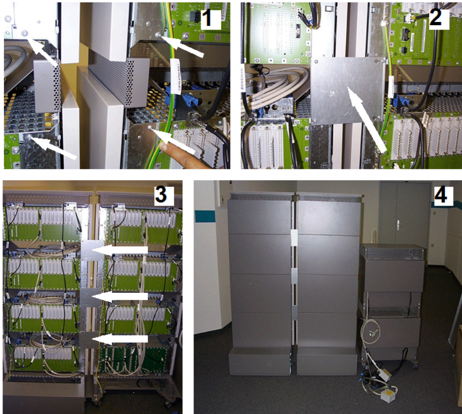
Figure 83: Installing the ground straps between the cabinets
