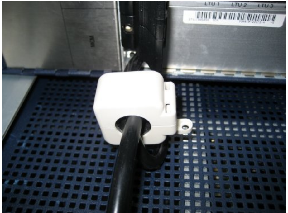
Figure 41: Closed ferrite core with AC cable
